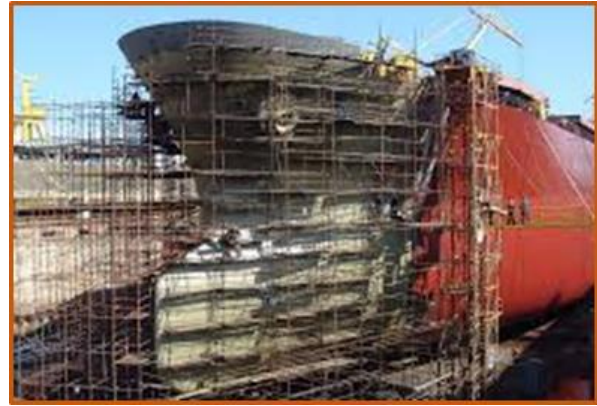
Ship hull construction
