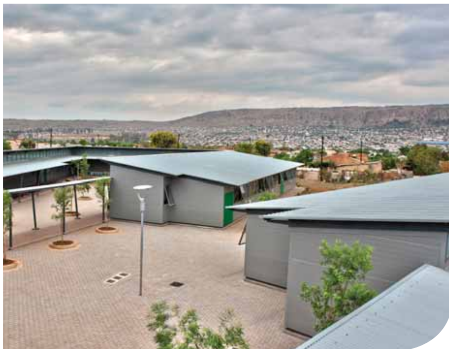
ArcelorMittal South Africa partnered with government in delivering the new Mandela Park Primary School to the Slovo Park community in Mthatha, Eastern Cape.
